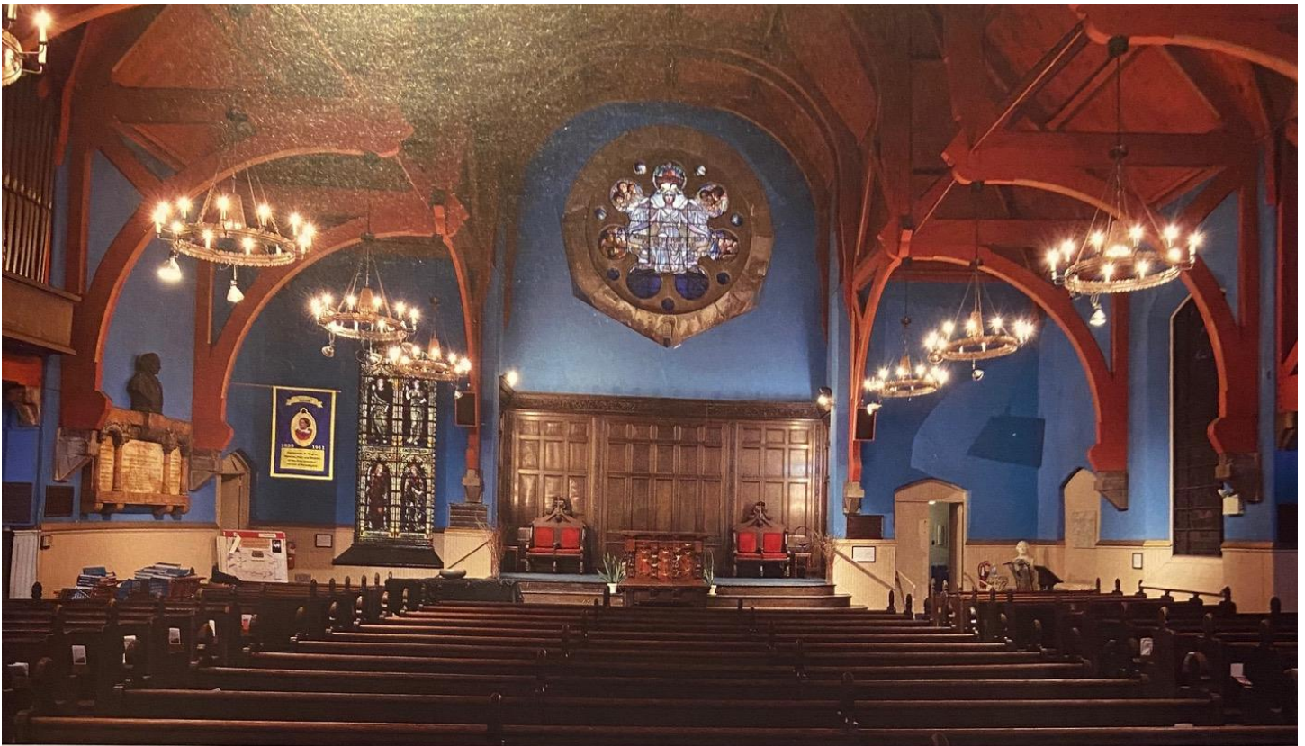
First Unitarian's arched trusses echo those of Rodeph Shalom and allow unobstructed sightlines in the broad sanctuary, as seen in this view from the front entry, across pews, and toward the chancel. PHOTO, PHMC
